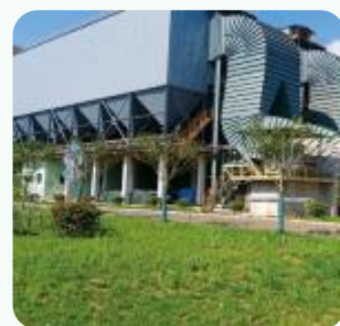
Secondary dust removal system in No.2 Steelmaking Plant
