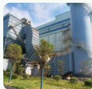
Blast Furnace ore tank bag dust removal system
